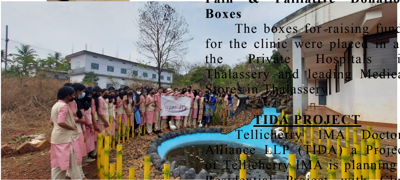
Water recycling plant built by the students(Pattanoor HSS)
